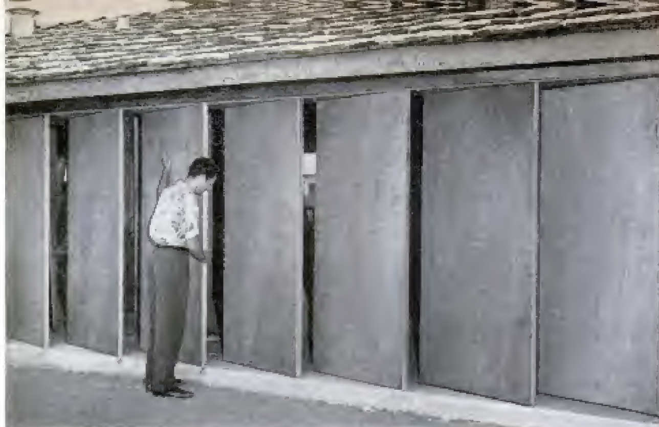
Bedroom wall consists of slab doors permanently set at a stagger. Movable glass panes will be between
